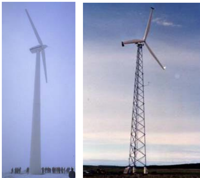
Figure 23 – Examples of horizontal axis wind turbines with a free-standing tubular tower (left) and a lattice tower (right)
