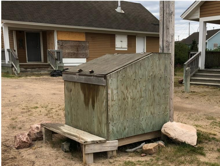
These Household Collection Boxes can be made from local wood in the Construction Shop. A log version of these boxes will be relatively easy to make—using primarily logs 2” in diameter. They will not require trucked-in OSB or plywood, will be bear-resistant, will look good, and will last a long time. By reducing the design’s dependence in imported plywood, they can be made more durable and easier to repair. This will also maximize local employment in construction.
