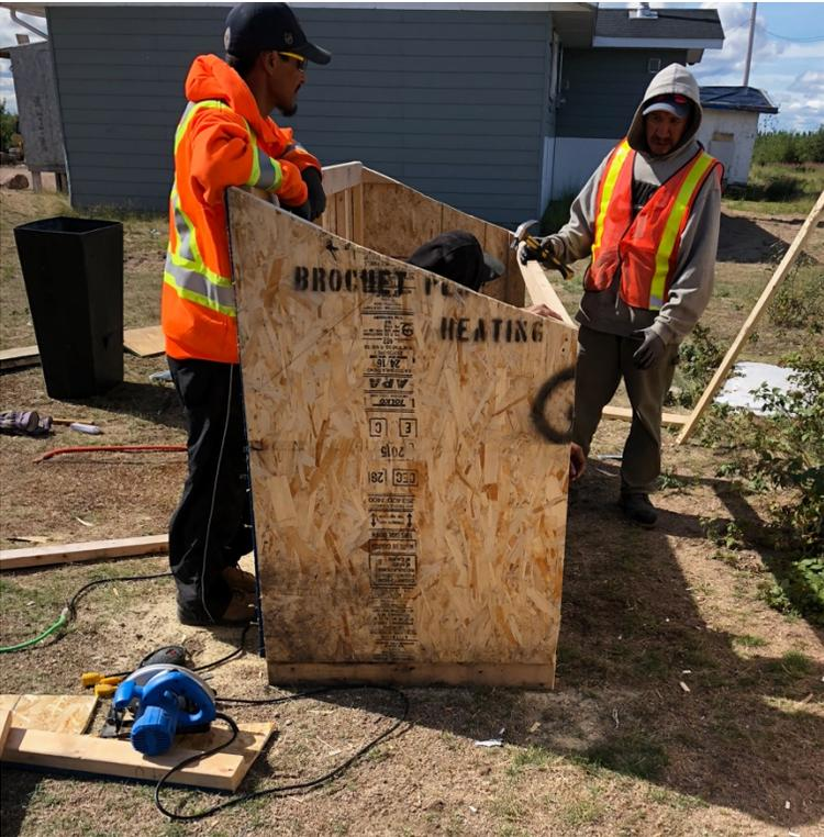
Figure 43: New Lid Design Using Salvaged Top of Derelict Appliance
