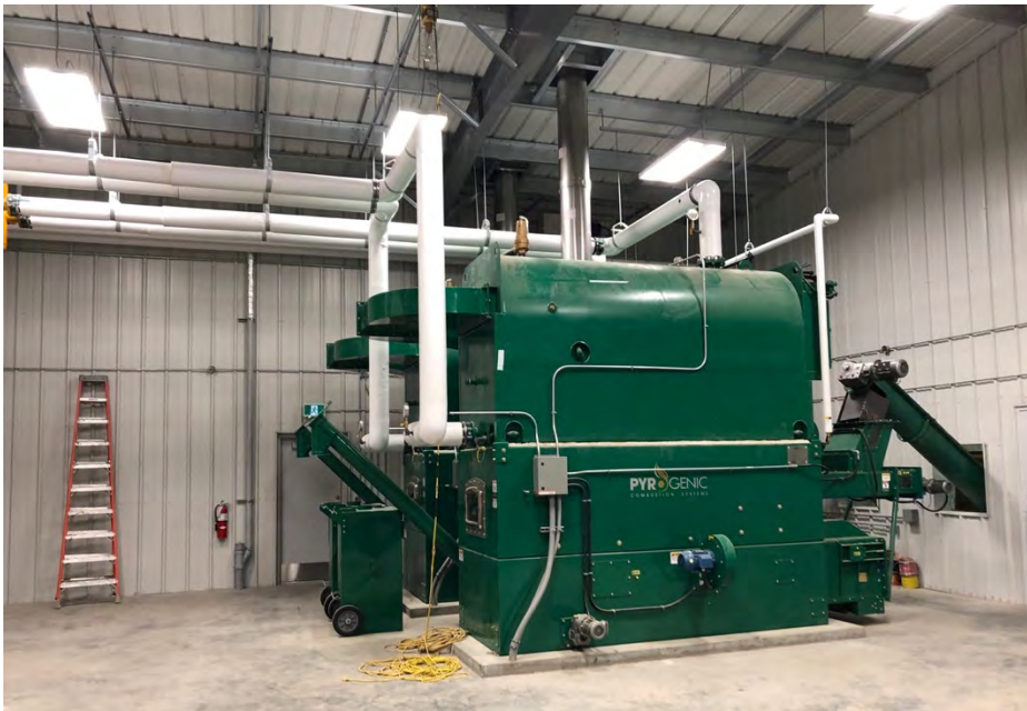
Figure 49: Biomass boilers using wood chips for fuel and heating a water/glycol mix distributed through a district energy system, Lac Brochet
