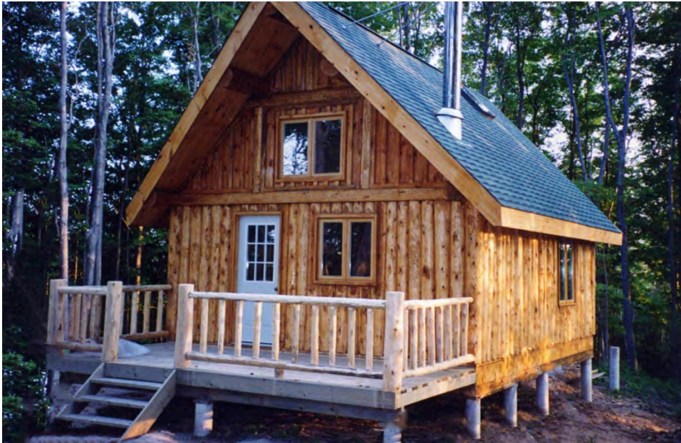
Figure 64: Example of vertical-log cabin construction 82
