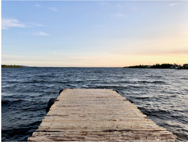
Figure 80: Dock Built with Small Logs at Lac Brochet
