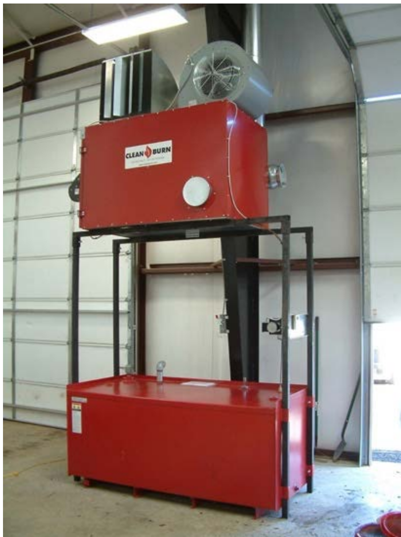
Figure 19 – Example of used oil handling and forced-air furnace system
