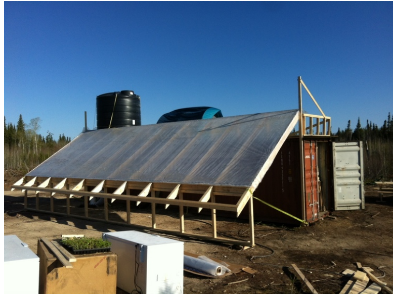
Figure 13: Garden Hill Greenhouse Exterior (Shown Under Construction)
