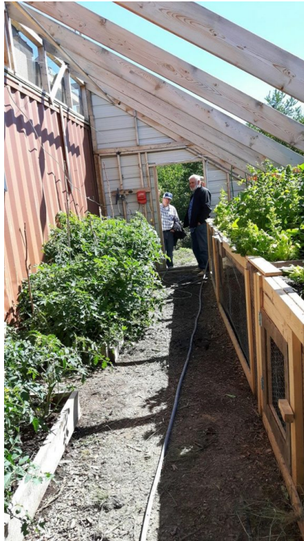
Figure 9: A Greenhouse Attached to the Side of a Shipping Container
