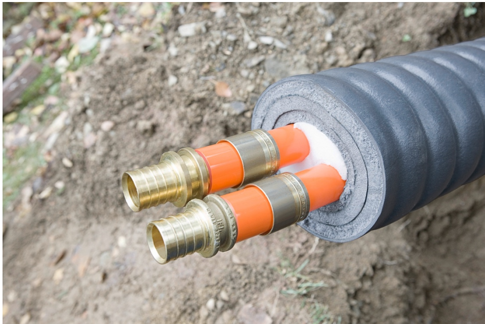
Figure 79. Close-up of Typical Insulated Underground Piping Connections 60
