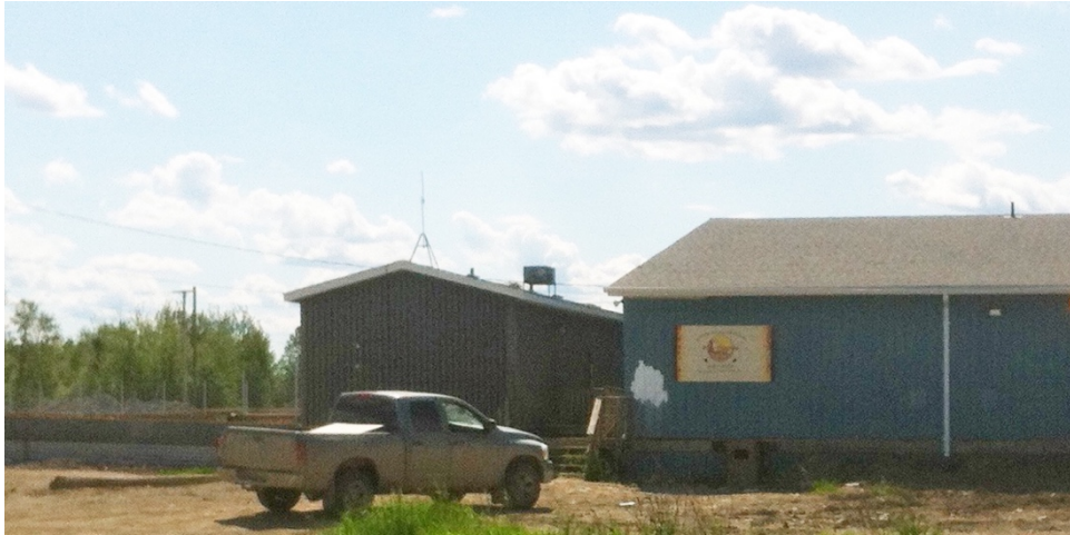
Figure 44. St. Theresa Point Ansinineew Government House
