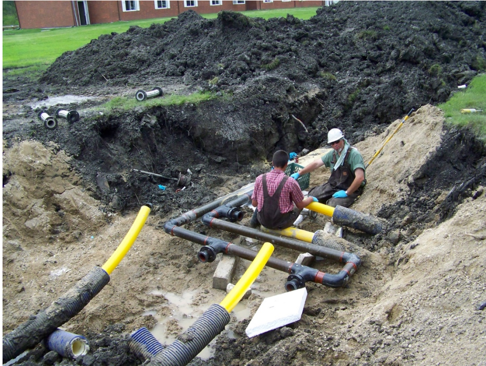
Figure 79. Close-up of Typical Insulated Underground Piping Connections 60
