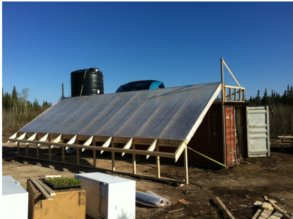
Figure 100. Garden Hill Greenhouse Exterior (Shown Under Construction)
